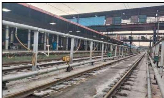
QUICK WATERING SYSTEM AT NEW DELHI
