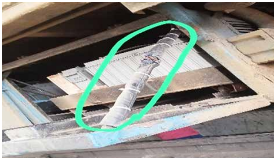
Provision of insulation sleeve on battery box cover leg
