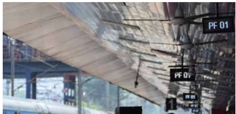
Coach Guidance System at Hazrat Nizamuddin Railway Station
